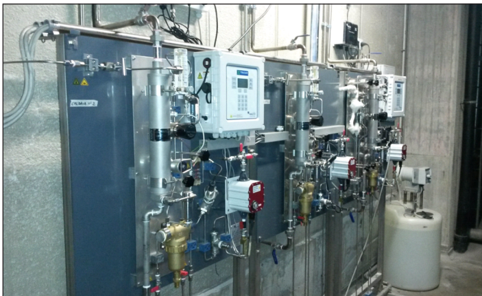
The new 3D TRASAR Boiler Technology units
