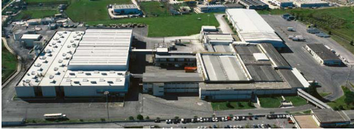
Figure 1: The Rieti Plant
