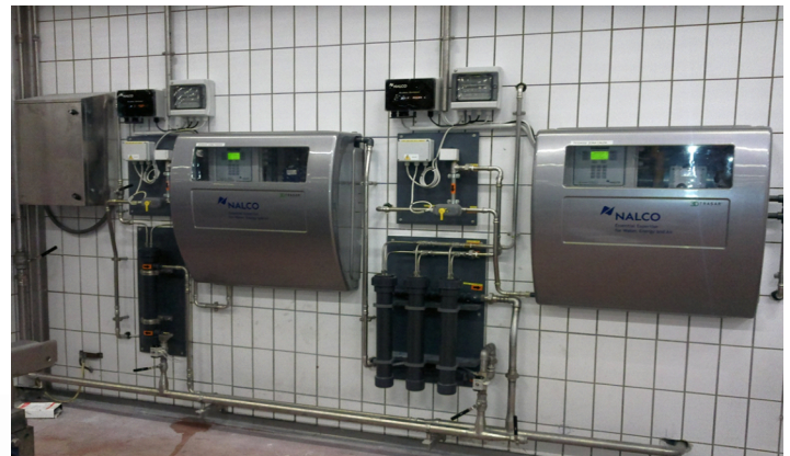
Nalco Water 3D TRASAR units in hot and cold legs of STORK hydrostatic sterilizer
